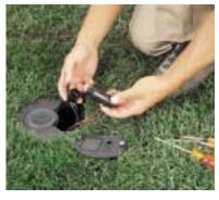
For the first time, access to the pilot valve, adjustable pressure regulator and solenoid is simple and easy.
